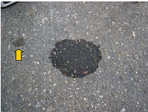
Oil Stain on porous, untreated concrete
